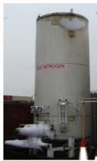
Perlite voids will slightly increase the natural boil off rate but as the vacuum remains in place it does not affect the safety of the installation.
