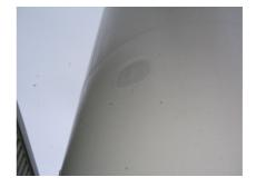
These frost spots do not affect the operation of the tank or the safety of the installation as the vacuum remains in place.
